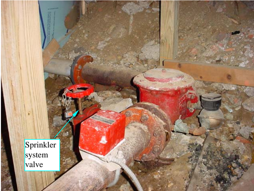
Sprinkler water Shut-off Located in Lobby Basement
